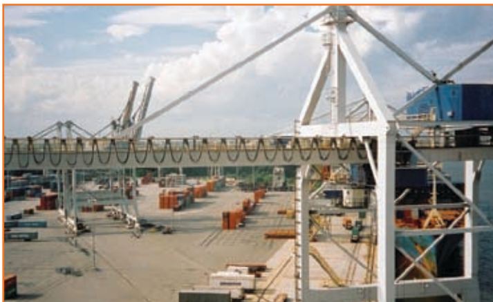
CONDUCTIX Festoon System on a Container Crane
