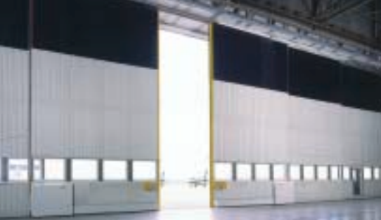
Electric hangar door with conductor rails and safety bumpers, protected height 52 ft
