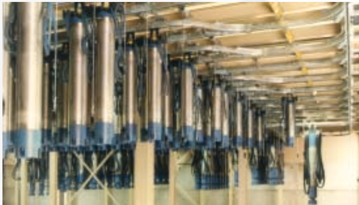
Overhead monorail with junctions for warehousing
