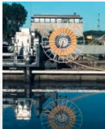
Motorized cable reel on a scraper in a sewage treatment plant
